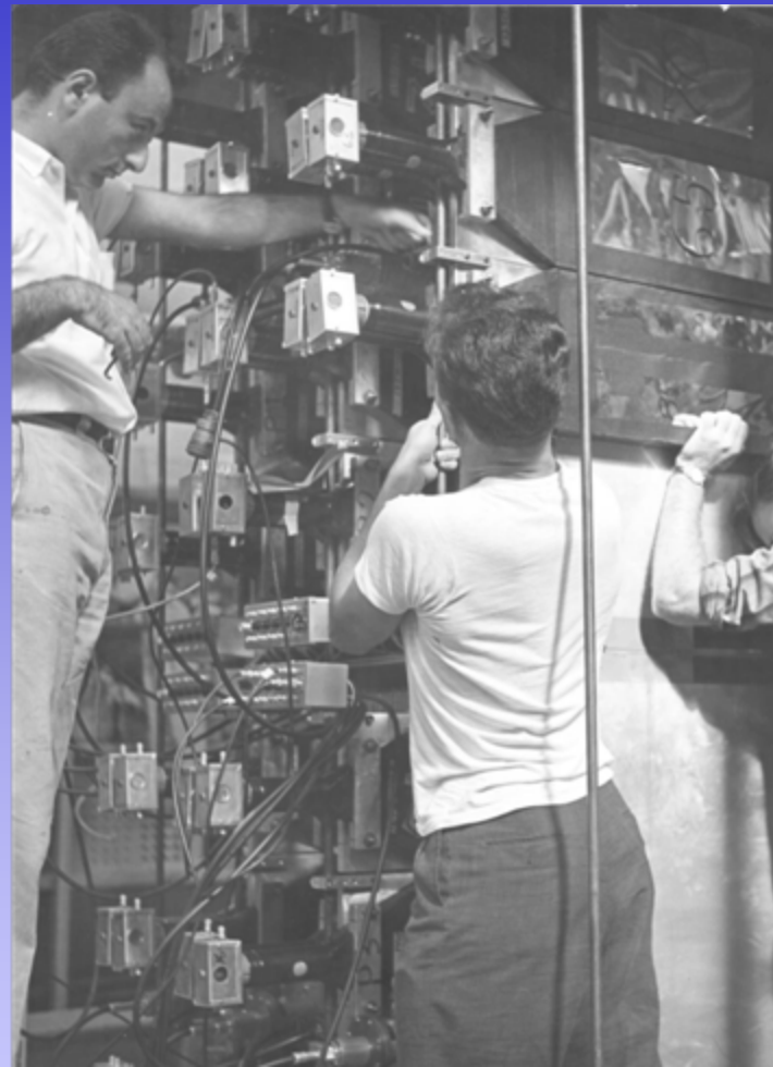
installing counters - Mel, Dino and 1/3 of (?)
