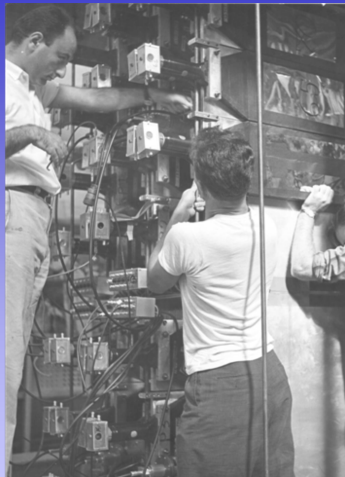
installing counters - Mel, Dino and 1/3 of (?)
